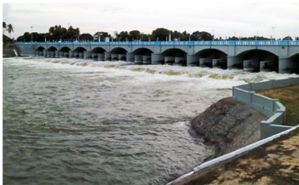
Figure 6. The Grand Anicut on river Cauvery Source: https://www.thecivilengineer.org/images/Manager/rpaigem/Front_View_Kallanai.jpg
