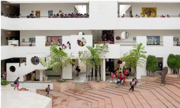
Fig. 7 Primary school in a neighborhood
