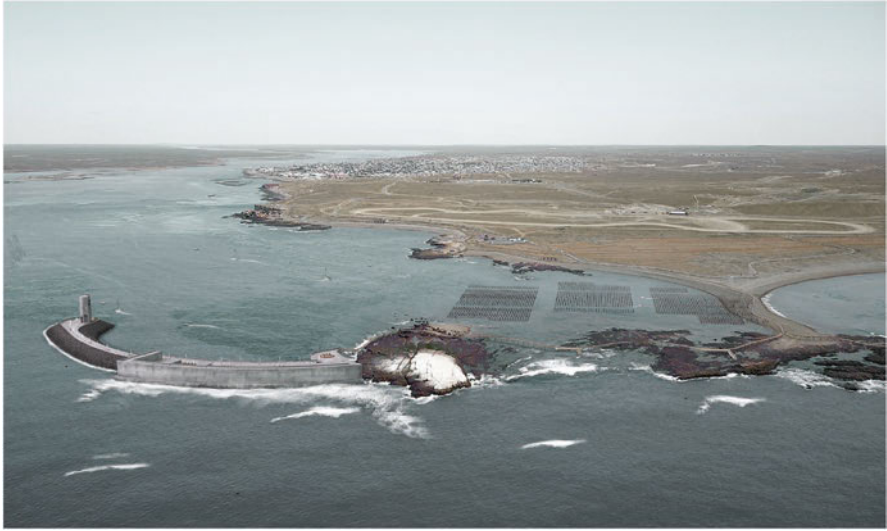
Fig. 3 Proposal for Puerto Deseado's Wave Energy Park, Patagonia. Panoramic view. Wave energy infrastructure that considers the geomorphology and directionality of waves. Creation of a semi-open and protected bay with productive and water sports programs. An urban-coastal vehicular and pedestrian connectivity links a series of scenic landmarks. (Image courtesy of Romagnoli-Pont-Serafini, designed in 2020)
