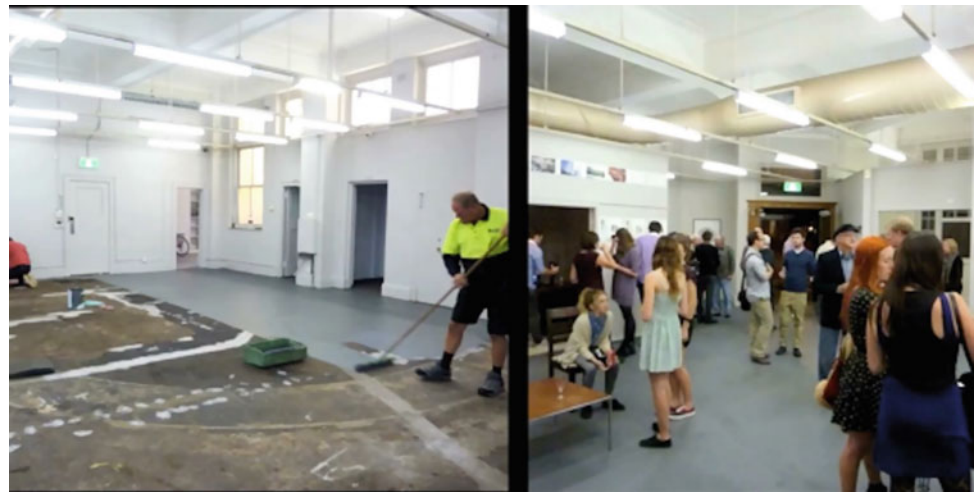
Fig. 9 Before and after the project in David Jones building (Renew Newcastle, 2018)
