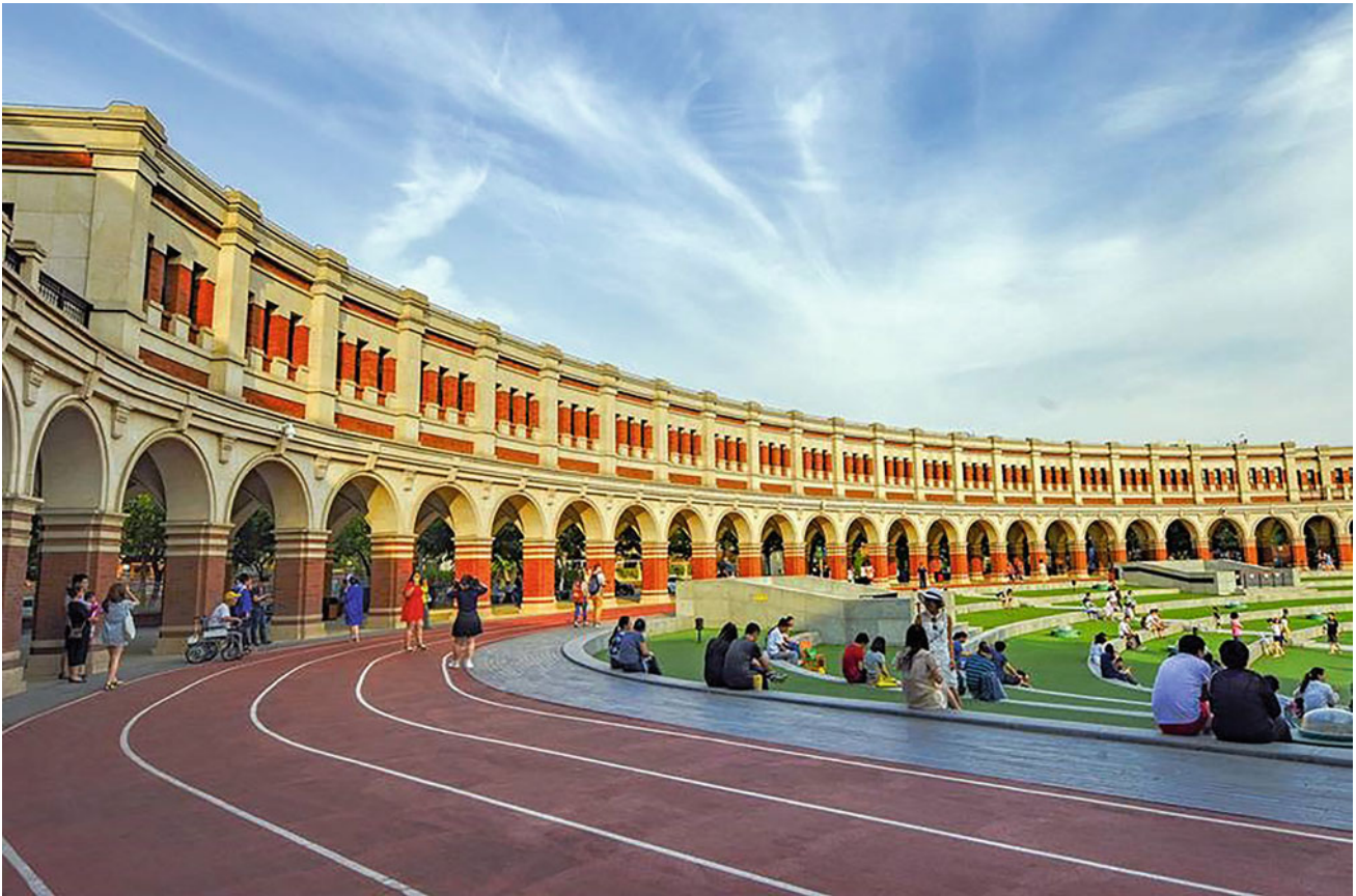
Fig. 13 (Right) Photo of Minyuan after rehabilitation. Photographer: Wenbin Yang
