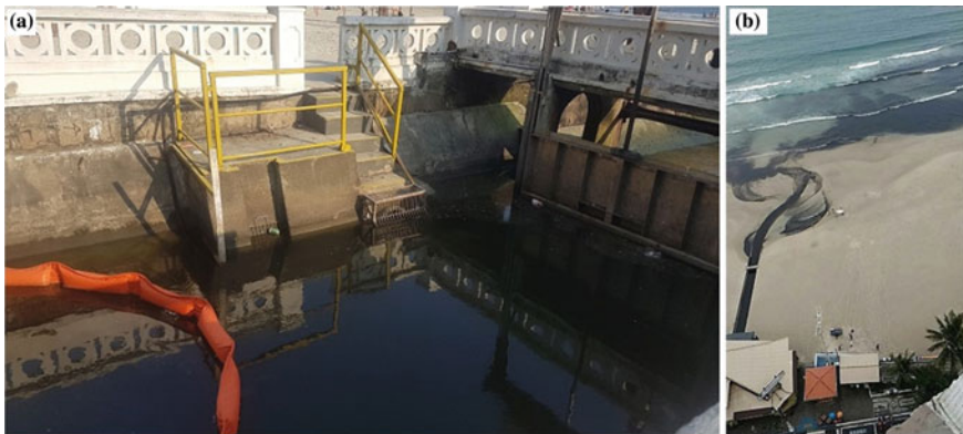
Fig. 6 a Content barrier system (configured in “U” shape), used to retain solid waste and other chemical and/or oily pollutants that are conducted into the urban drainage channels in Santos, Brazil; b Accidental sewage leak in Pitangueiras beach, Guarujá, Brazil (in 2018), conducted to the sea through urban drainage channels. Source Personal archive
