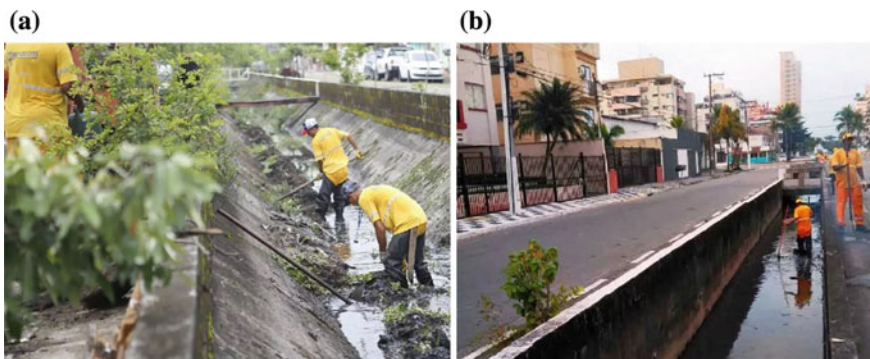
Fig. 3 Services of silting (a) and cleaning (b) performed by the city hall of Guarujá in the urban drainage channels of Enseada, Guarujá, São Paulo coastal zone, Brazil. Source Personal archive
