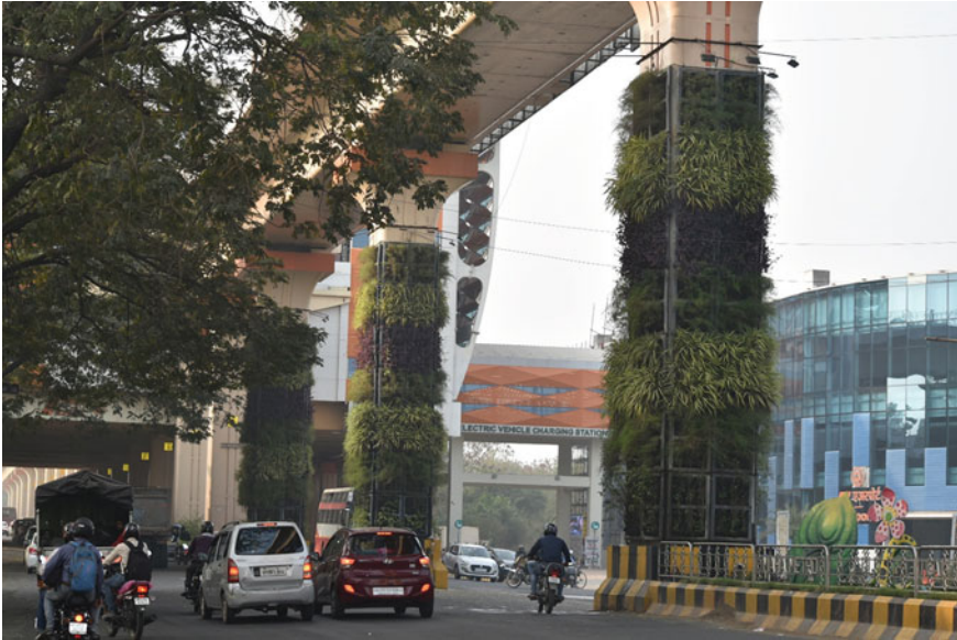
Fig. 2 Vertical greenery on the pillars supporting the Nagpur Metro line (India, © Deepak Dhyani)
