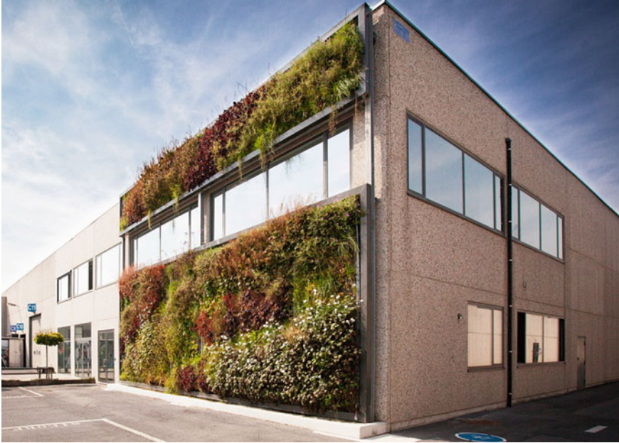
Fig. 5 A green wall on an office building (©Sioen Industries)
