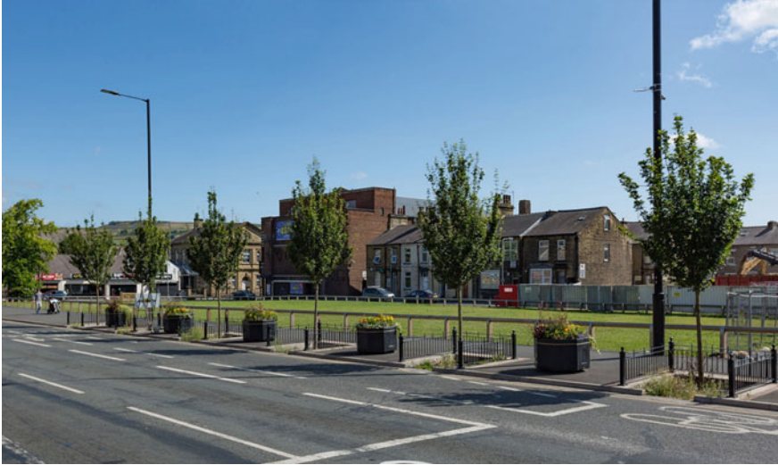
Fig. 8 Trees planted in tree pits to prevent road runoff (North Street, Keighley, Yorkshire, UK. © GreenBlue Urban)
