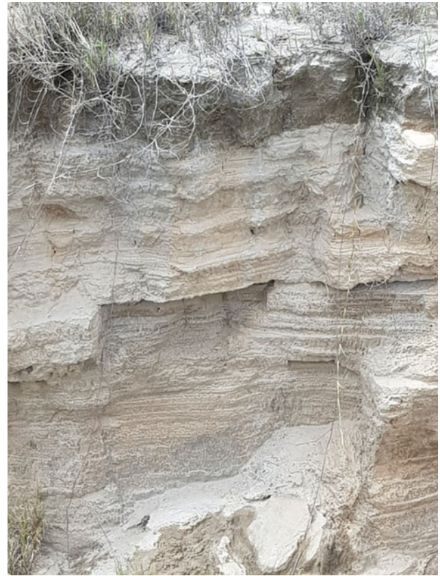
Fig. 19.5 Protic Regosol (Geoabruptic) developed on Monarch gold mine tailing dam in Francistown. Depth ~100 cm
