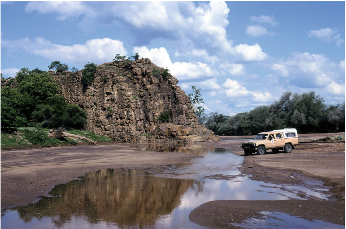
Fig. 16.7 View of Solomon's Wall in the lower part of the Motloutse River, Botswana. Photo Frank D. Eckardt
