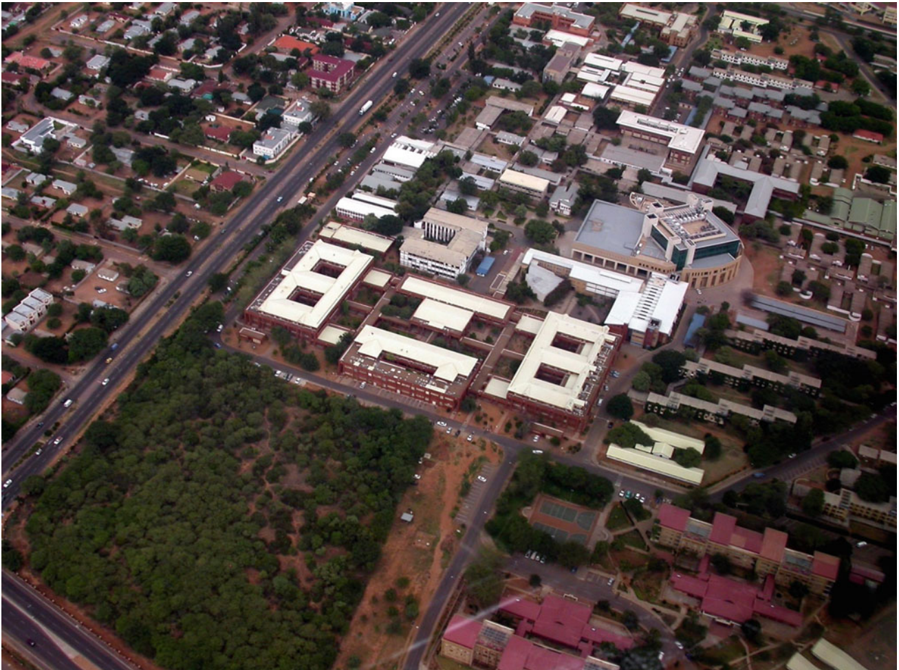
Fig. 1.9 Aerial view of University of Botswana, Science Block, Environmental Science and Geology Departments on the southside of campus (Photo: Frank D. Eckardt)
