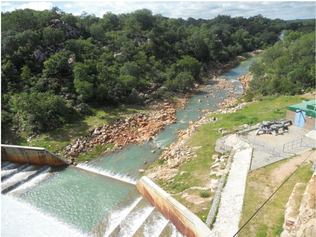
Fig. 17.10 Ntimbale dam spilling in 2011
