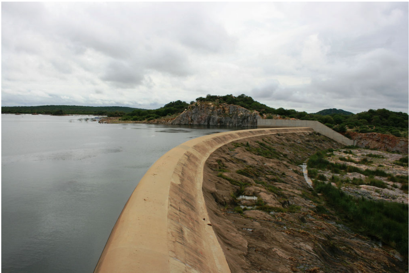
Fig. 17.5 Letsibogo Dam feeds into the North–South Carrier (NSC) and can supply water to Gaborone some 300 km away
