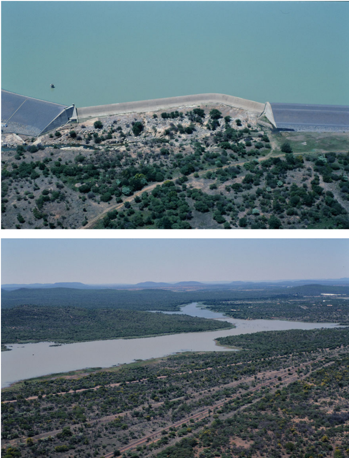
Fig. 17.2 Gaborone Dam the oldest in the country as been expanded by raising the wall (top) and extending it with a second wall at Notwane (bottom). Note the changing alignment and abandonment of roads and
