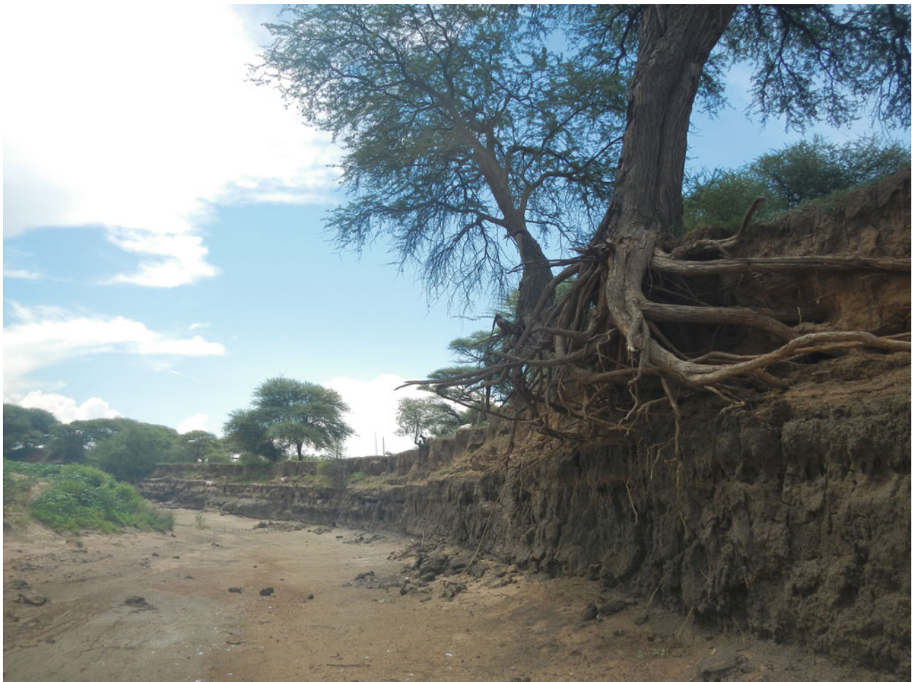
Fig. 17.7 Bank erosion on the Metsemothabe River just outside Gaborone
