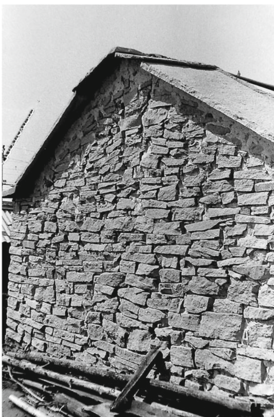
Fig. 5 A shed with walls and roof of the limestone of the stone slabs. The village of Chernorechye, Troitsky district, Chelyabinsk region. The ban on the use of wood for construction contributed to the emergence of such architecture. Pay attention to the roofing material—stone slabs. Photo by Nikolai B. Vinogradov
