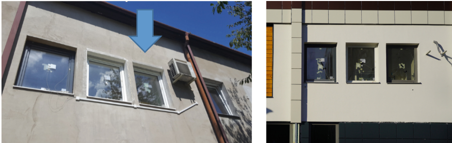
Fig. 1. Outer view on the built-in windows before and after façade renovation.
