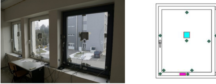
Fig. 2. Inside view in the room with test windows. Visible positions of sensors and heat flux plates. Sketch of window with marked position of sensors.
