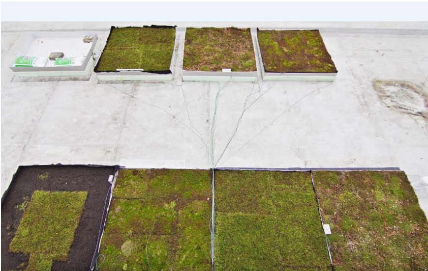
Fig. 2. View of different green roof compositions: upper row for measuring the rainwater retention, bottom row for measuring the temperatures.
