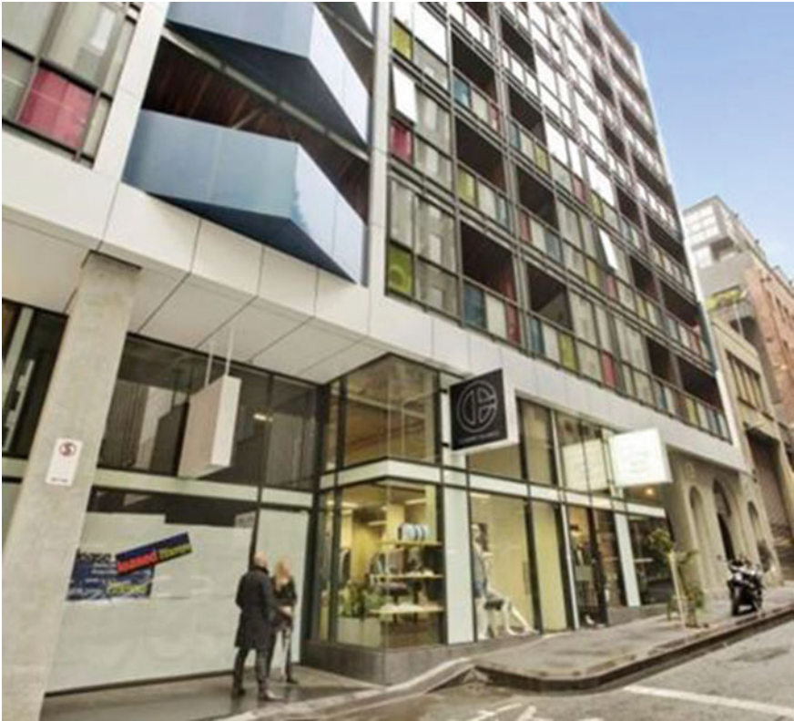
Fig. 5.13 Modular building for offices (Navaratnam et al., 2019)
