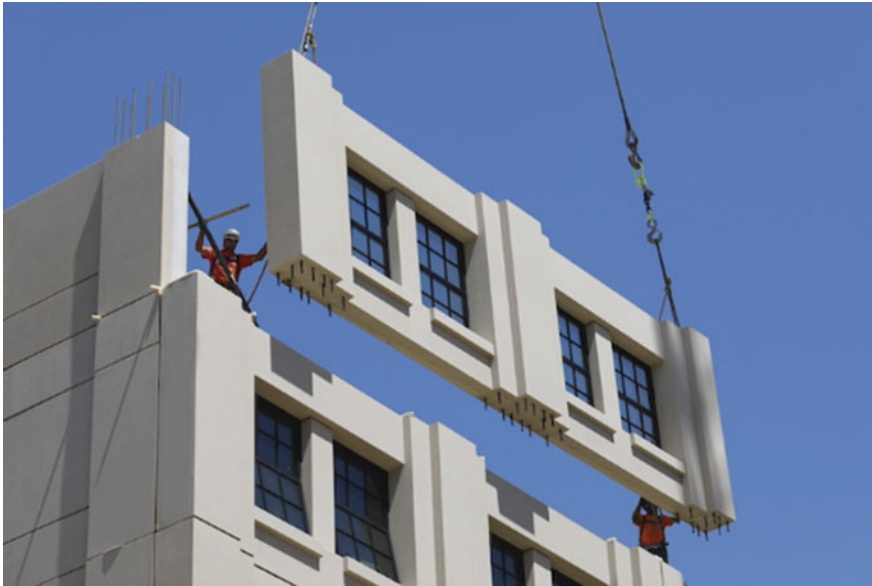
Fig. 5.1 An exterior wall panel (John, 2020)
