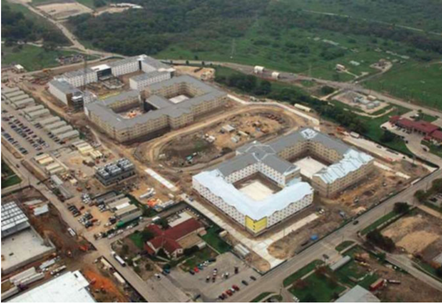
Fig. 5.15 Fort Sam Houston medical education and training complex in San Antonio, Texas (Ankit, 2016)
