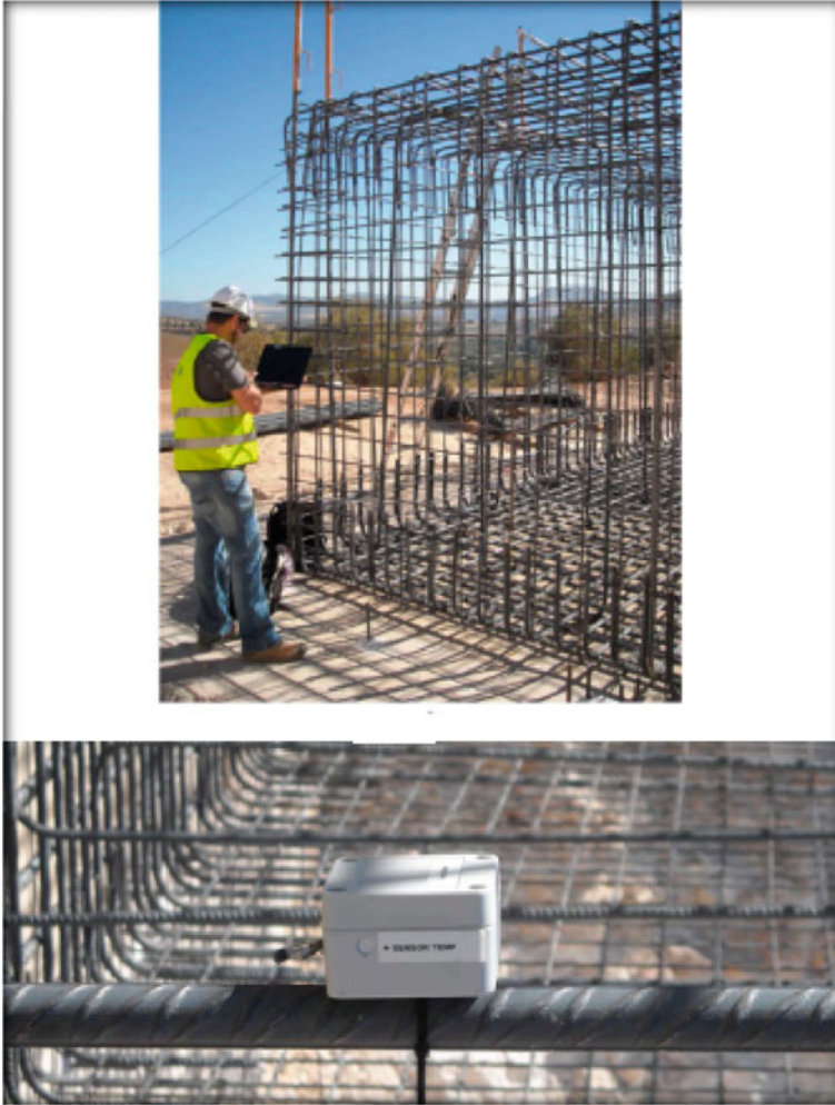
Fig. 8.14 A sensor connected to a cast iron (Cabezas et al., 2018)
