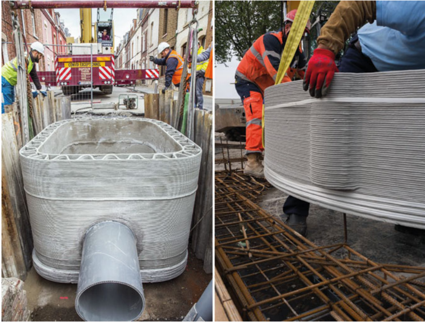
Fig. 6.12 3D-printed stormwater collectors (GaudilliEre et al., 2018)
