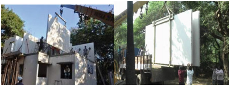
Fig. 5.2 Panels assemble on site (Anuradha & Dhawade, 2015)
