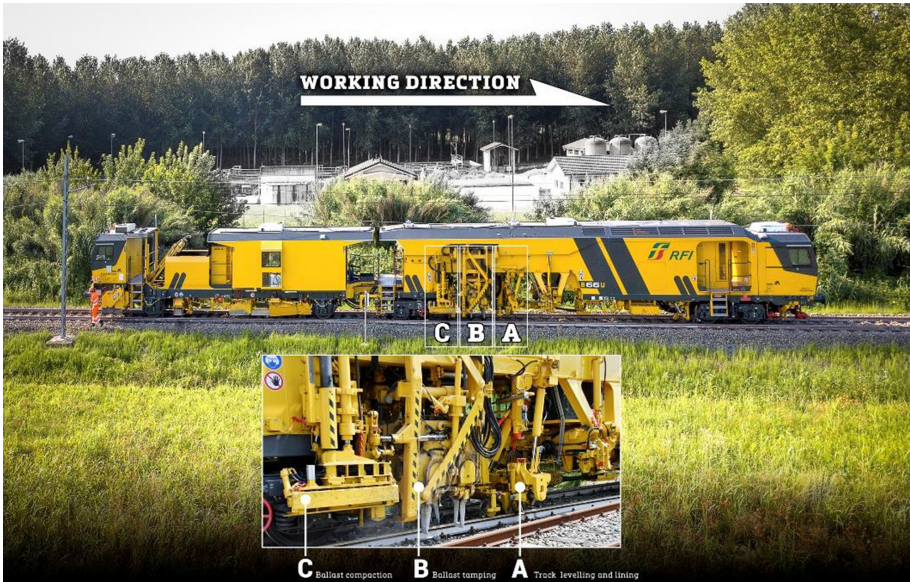
Fig. 1. Ballast tamping machine in operation
