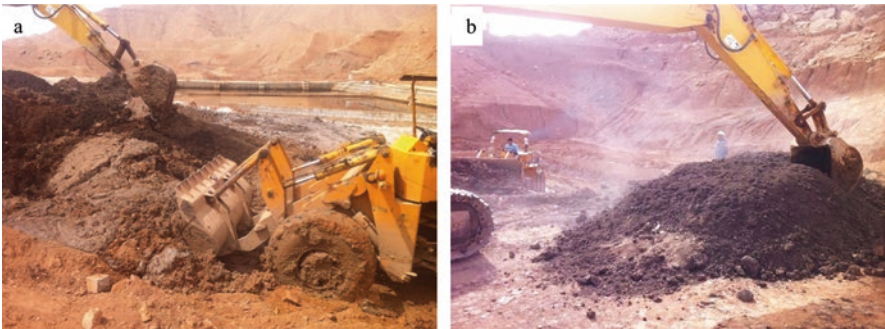
Fig. 4.8 Biological drying of cuttings and solids (Naft Sefid, Shushtar County, Khuzestan province, Iran, 2019) : (a) Absorbing water by organic materials; (b) evaporation of water
