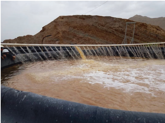
Fig. 4.5 Shower operation over ponds. (Naft Sefid, Shushtar County, Khuzestan province, Iran, 2019)
