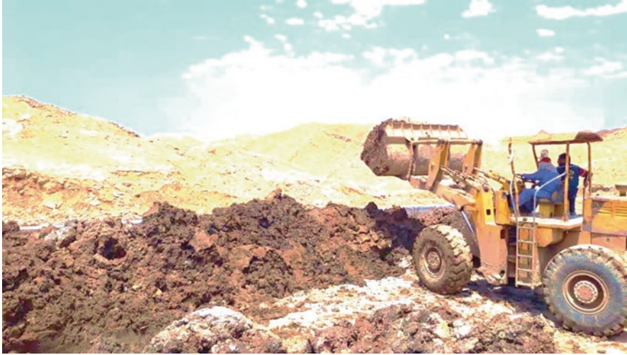
Fig. 4.9 Pile composting of drilling oil and gas well solid wastes. (Naft Sefid, Shushtar County, Khuzestan province, Iran, 2019)
