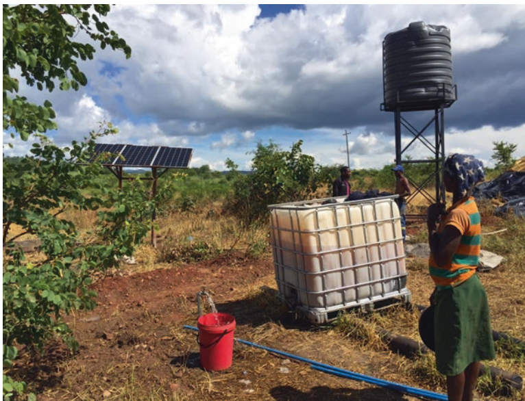
Fig. 10.2 Solar-powered boreholes integrating community and business needs for safe development. Source: Blue Chip Engineering Ltd. Zimbabwe (2021)
