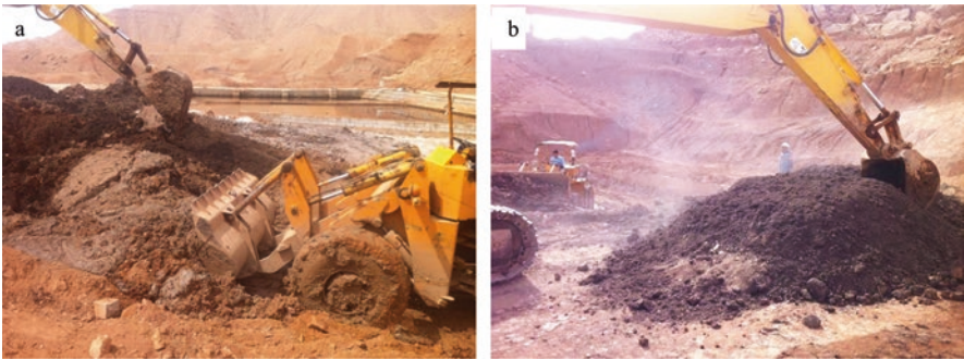
Fig. 4.8 Biological drying of cuttings and solids (Naft Sefid, Shushtar County, Khuzestan province, Iran, 2019) : (a) Absorbing water by organic materials; (b) evaporation of water
