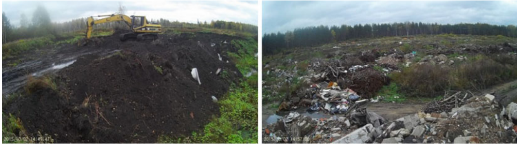
Fig. 15.6 Site V: Ash disposal area on primitive brownfield soil
