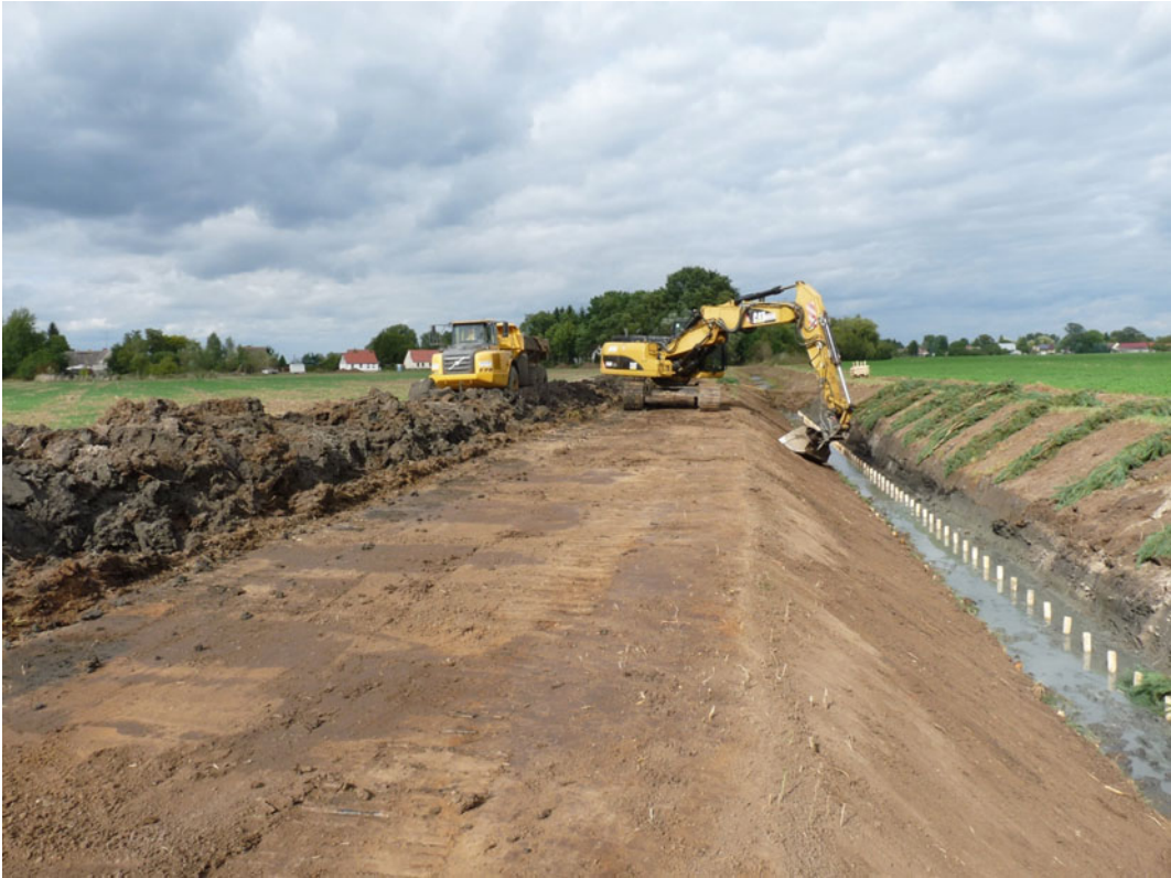
Fig. 2.9 Ditches for land drainage and other land reclamation constructions are primarily physical impacts in to soils of wetlands. They initiate physical and biological soil reclamation processes. Their positive effect
