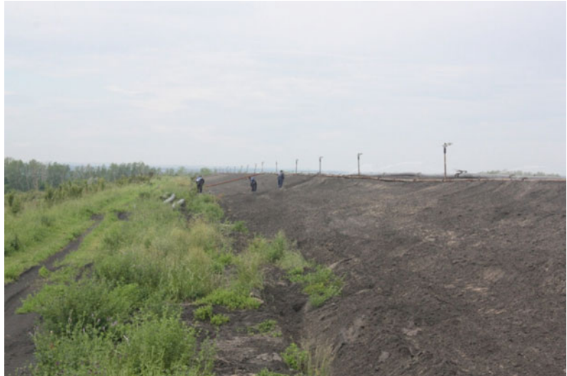
Fig. 26.5 Phytoremediation of fly ash dump in the passive fly ash dump of “Nikola Tesla B” thermal power plant, Obrenovac, Serbia (TENT B) (Photo by L. Maričić)
