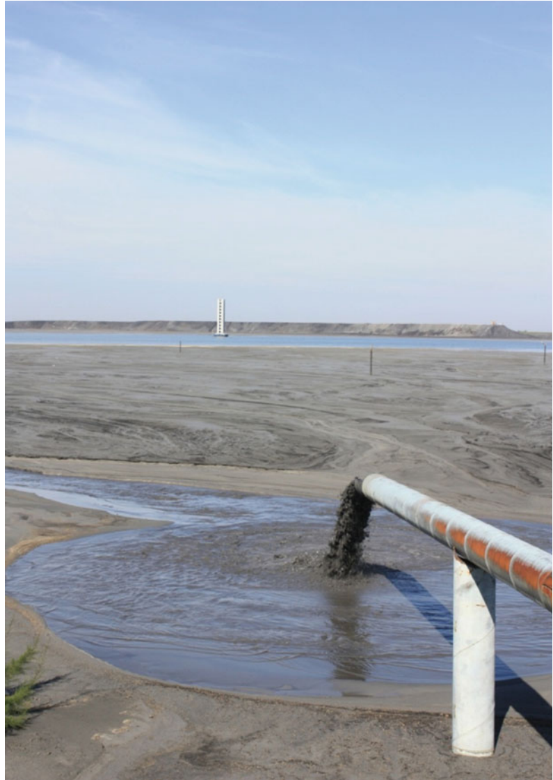
Fig. 26.2 Active surface fly ash dump at the “Nikola Tesla A” thermal power plant (TENT A), Obrenovac, Serbia (Photo by L. Maričić)
