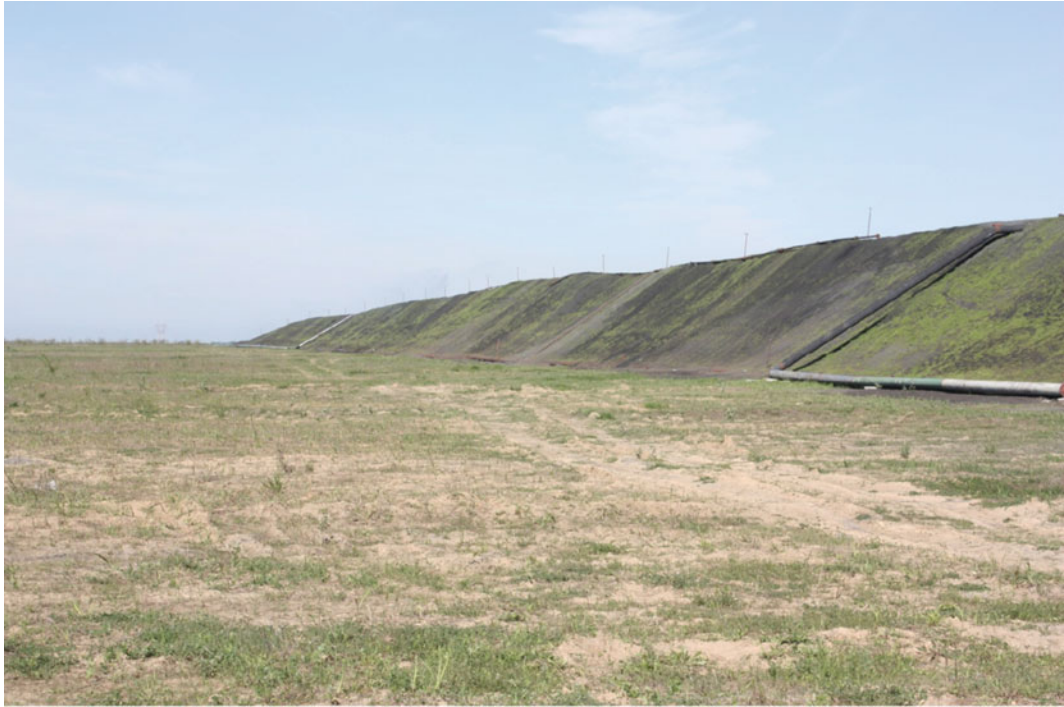
Fig. 26.3 Passive fly ash dump at the “Nikola Tesla A” thermal power plant (TENT A), Obrenovac, Serbia (Photo by L. Maričić)
