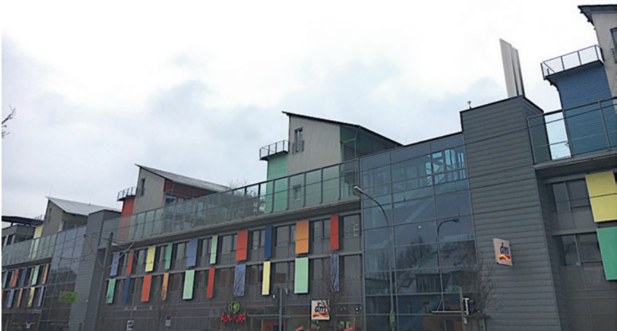
Fig. 2.6 Fully roof-integrated BIPV design at the Plus Energy Settlement, Freiburg, Germany, (Aelenei, L., Waldren, D., Aelenei, D., Cúbi, E., Wittchen, K., Kim, J., (2017). Net ZEB case study buildings, measures and solution sets. In: F. Garde, J. Ayoub, L. Aelenei, D. Aelenei, and A. Scognamiglio, ed., Solution Sets for Net Zero Energy Buildings, Feedback from 30 NZEBs worldwide , 1st ed. Wiley-Ernst & Sohn. ISBN 978-3-433-03072-1). (Photos by Laura Aelenei)
