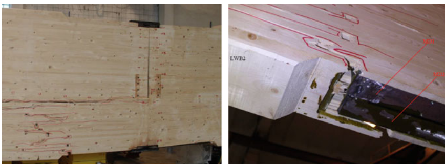
Fig. 12 General view of the failure of the specimen joint
