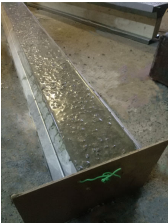
Fig. 9 Concreting the side segments of the steel pillar
