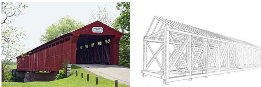
Fig. 1 Elden Bridge, built in 1860 [4]
