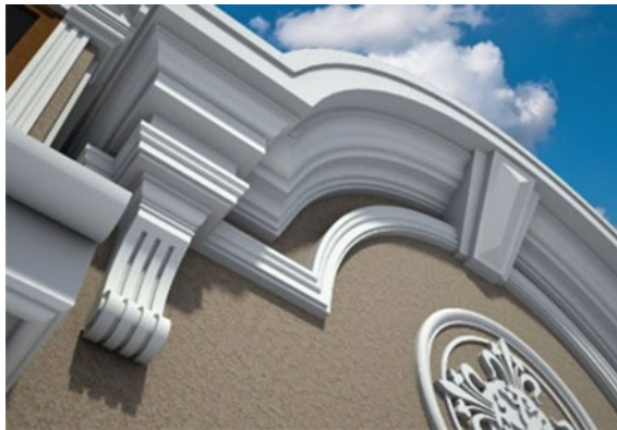
Fig. 7 Residential house. Fragment of the facade. The texture affects the lighting. The intensity of the illumination of the object decreases with the increase of the roughness and unevenness of the body surfaces. Sometimes the irregularities on the surface of the form reach such dimensions that their illumination drops sharply due to the appearance of their own shadows and those that fall on the surfaces themselves. The luminance of the surface depends on its color. White strongly reflects light, and black, on the contrary, actively absorbs it [15]
