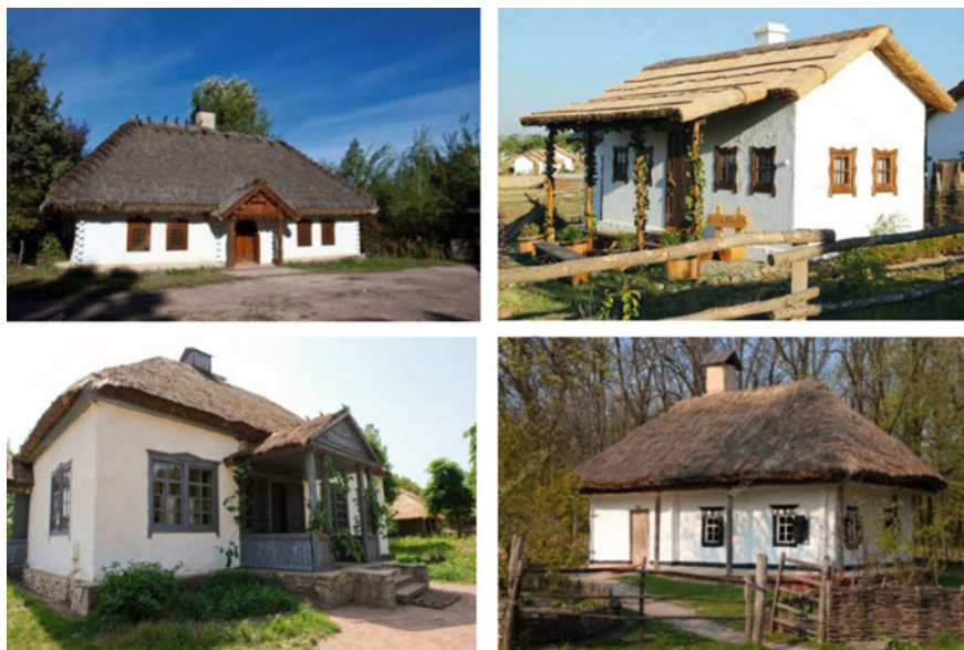
Fig. 1 In the middle of the twentieth century, a porch covered with a gabled roof with a pediment became widespread. The porch (a small canopy over the entrance) was supported by light wooden supports
