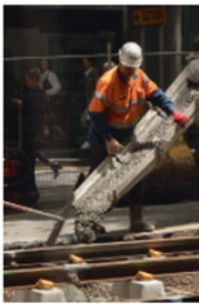
“construction worker in orange safety vest is working on road”
