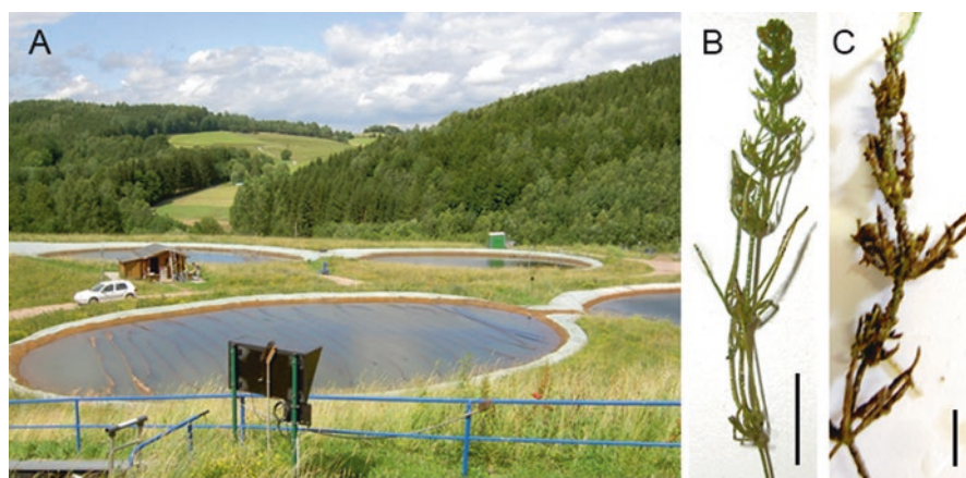
Fig. 9.20 Bioremediation ponds in Pöhla (Boojum and Wismut, GmbH), Germany (a). Scale-up of the pilot test system at Pöhla (b). Non-encrusted C. vulgaris from the unpolluted reference site near the bioremediation ponds. (c) Heavily encrusted C. vulgaris from the bioremediation pond, scale bar = 1 cm. (Photographs: H. Schubert)
