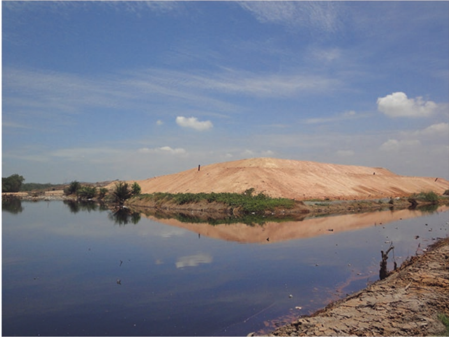
Fig. 8.9 Leachate collection pond prior to treatment
