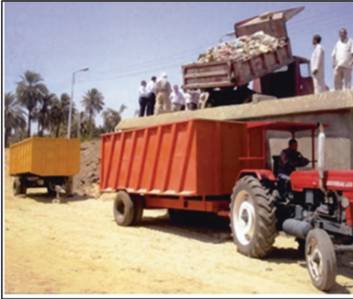
Fig. 3.27 Platform station invert [30]
