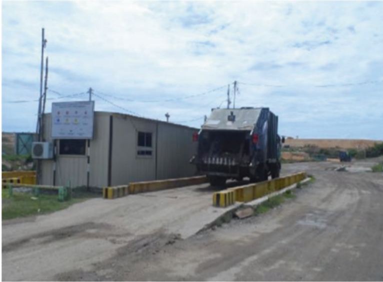
Fig. 4.8 A typical weighbridge system
