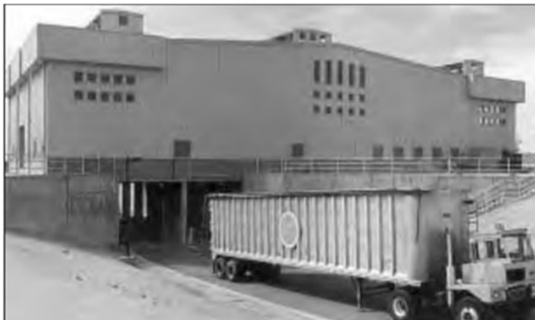
Fig. 3.28 Stationary compactor system in a combine transfer station invert and put [73]
