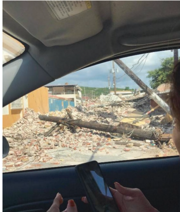
Fig. 2 Electrical poles damaged by earthquakes in Guayanilla, Puerto Rico (Photo source: Katherine Morales, 2020)
