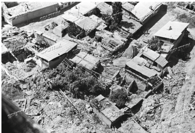
Fig. 5 Damaged individual residence after 1966 event (01.05.1966 photo by G.Zelma)
