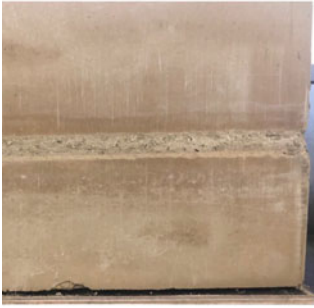
Mortar between CEB
