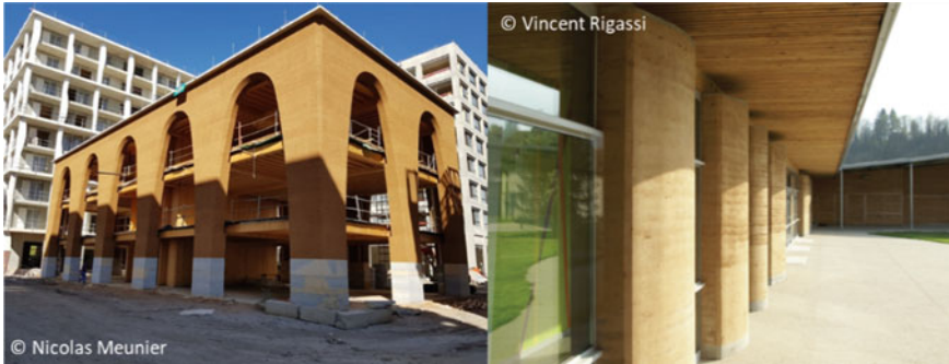
Fig. 1.6 Examples of modern earthen constructions
