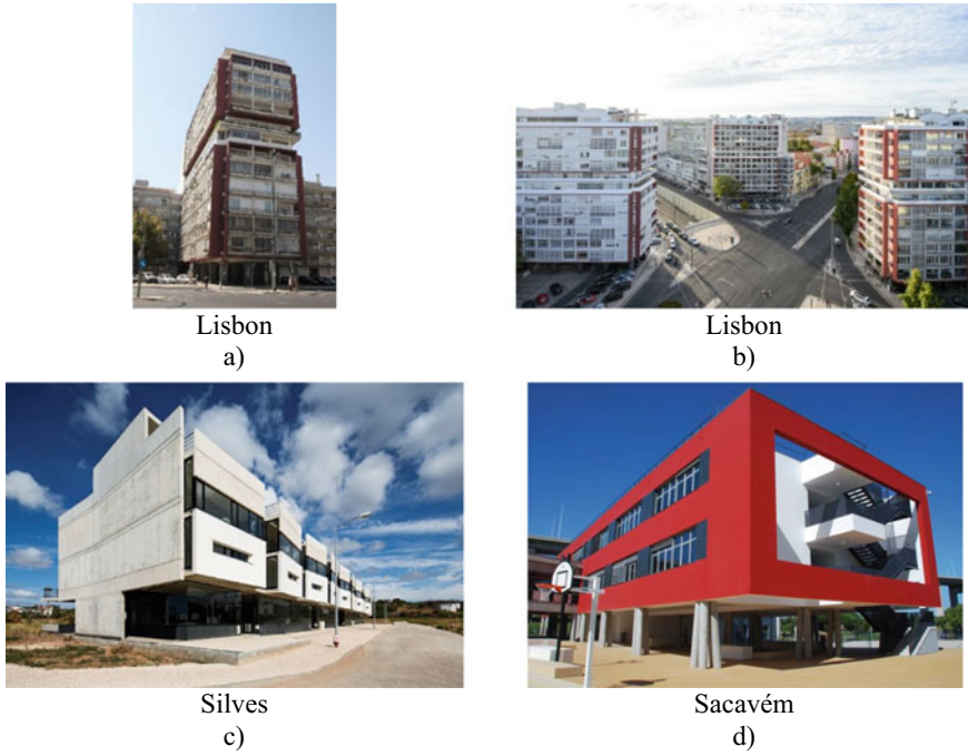
Fig. 5 Examples of buildings with soft-storey configuration located in Portugal: a 11-storey building, b general view of 11-storey building structures, c 4-storey building and d school building
