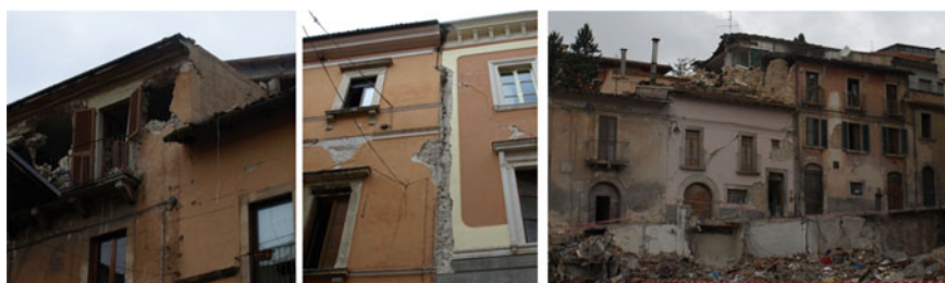
Fig. 4 Examples of damages observed after the L'Aquila (2009) event, due to interaction between adjacent buildings within an aggregate (Photos: A. Penna)
