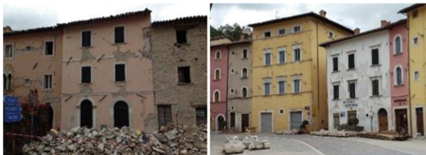
Fig. 3 Examples of global in-plane seismic damage to building aggregates, observed after the Central Italy sequence of 2016–2017 (Photos: A. Penna)
