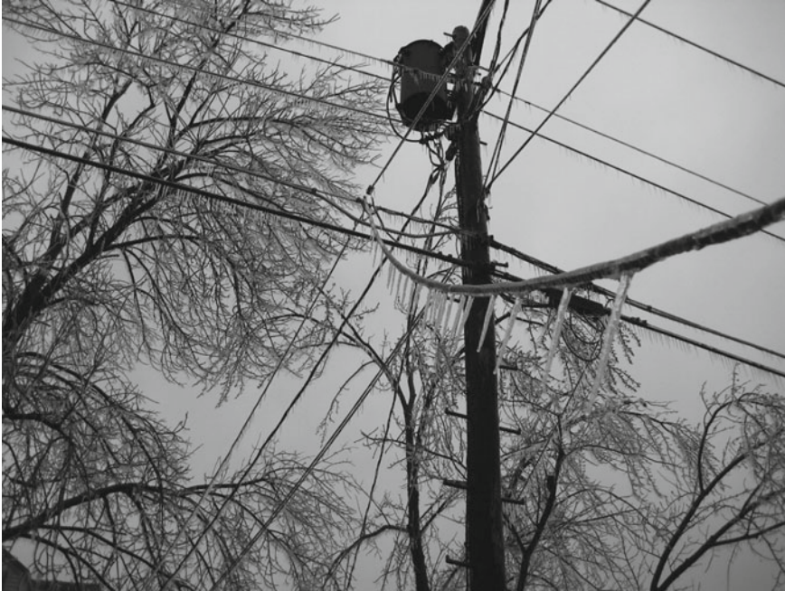
Fig. 8.2 Atmospheric icing of the overhead power line. Title: IMG_0337. Author: KOMUnews. Source https://flic.kr/p/4cEson . License: CC BY 2.0
