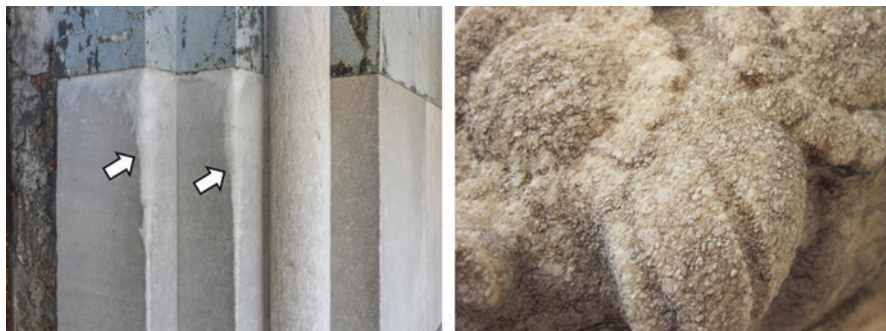
Fig. 1.4 Left, rounding along the edges of blocks of fine-grained Crevoladossola marble (dolomitic marble, Monza Cathedral, Italy) due to the erosive effect of water runoff. Right, roughening of the sculpted decorative element of Candoglia marble (medium- to coarse-grained calcitic marble, Milan Cathedral, Italy) due to the combined action of rain and thermal dilation
