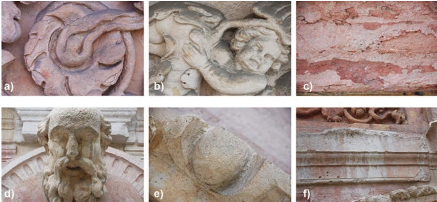
Fig. 1.7 Photographic documentation of characteristic deterioration patterns in sheltered conditions (a, crust; b, deposit; c, exfoliation) and in areas subjected to the rain runoff (d, erosion and encrustation; e, pitting; f, bleaching)
