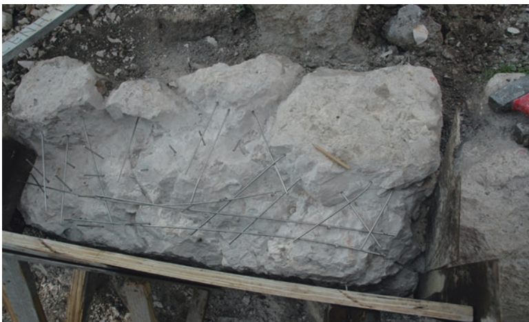
Fig. 7.3 Stainless steel rods embedded in the stone body before repairing, from [26]
