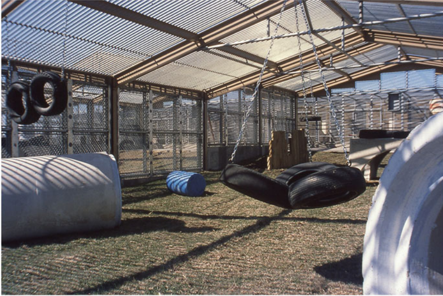
Fig. 2 Large outdoor exercise structure at the Southwest Foundation for Biomedical Research, San Antonio, Texas in 1989. Photo courtesy of Dr. T.M. Butler
