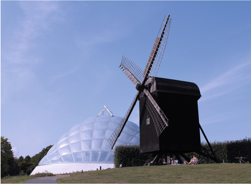
Fig. 12 Finished building in context (© Paul Shepherd)
