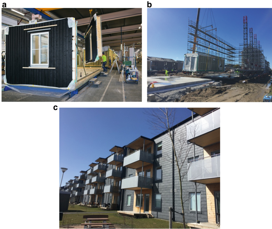
Fig. 5 a Module production at BoKlok factory, b on-site module assembly, c finished BoKlok housing
