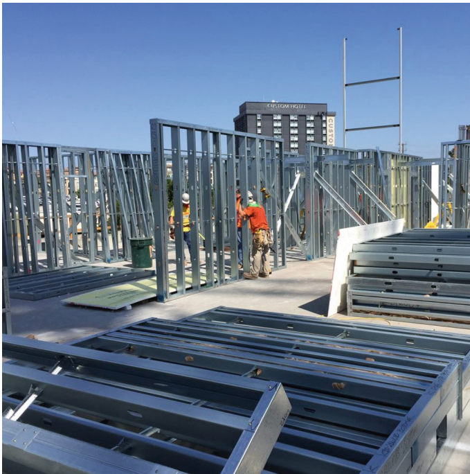
Fig. 9 Workers install one of DBC’s wall panels
