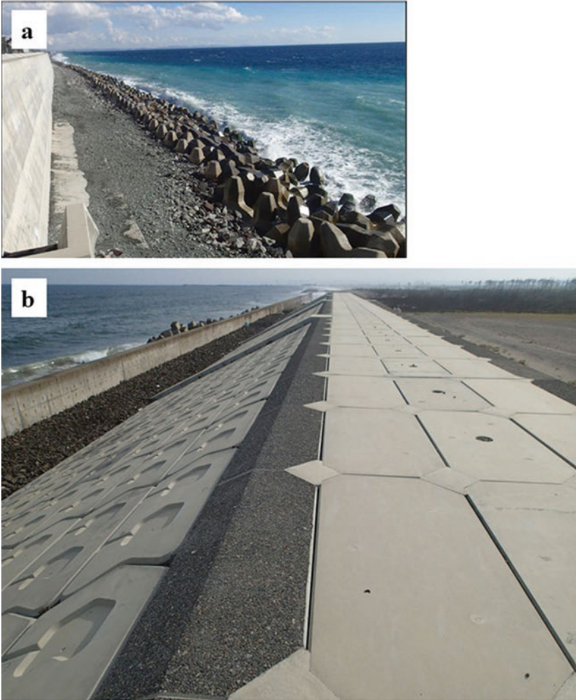
Fig. 1 Some views of coastal Japan. (a) typical artificialized beach along the coast of Japan; (b) giant sea wall construction after the Great East Japanese Earthquake of 2011
