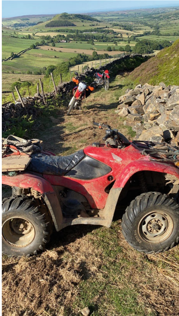
Fig. 2 Access is difficult for some walls. Fryup North Yorkshire (Source: The author)
