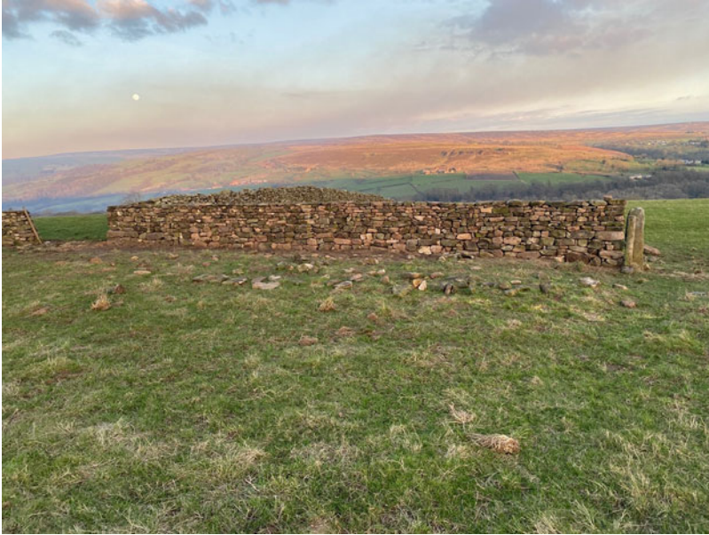
Fig. 6 A completed section of wall (Source: The author)
