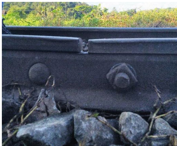
Fig. 7 Side view of the step joint
