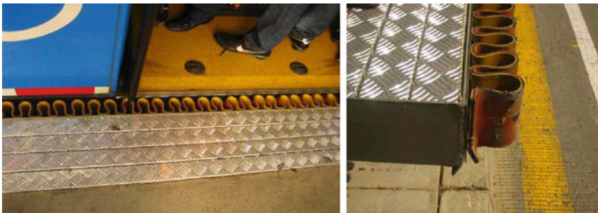
Fig. 11 Corrugated platform edge (Rickert 2010)
