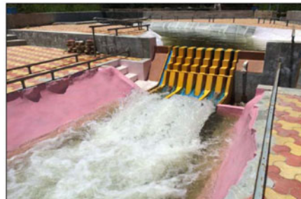
b) Gated operation of spillway
