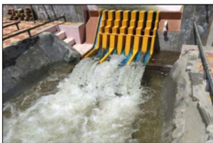
a) Ungated operation of spillway
