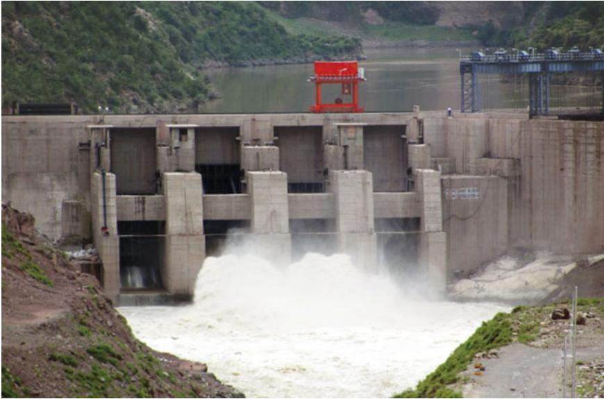
Photo 14.2 Downstream view of spillway Commissioned Uri-II H. E. Project, Jammu and Kashmir ( https://www.hccindia.com/markets/hydro-power )
