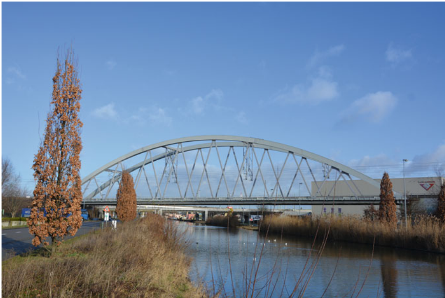
Fig. 10 Railway bridge KW51
