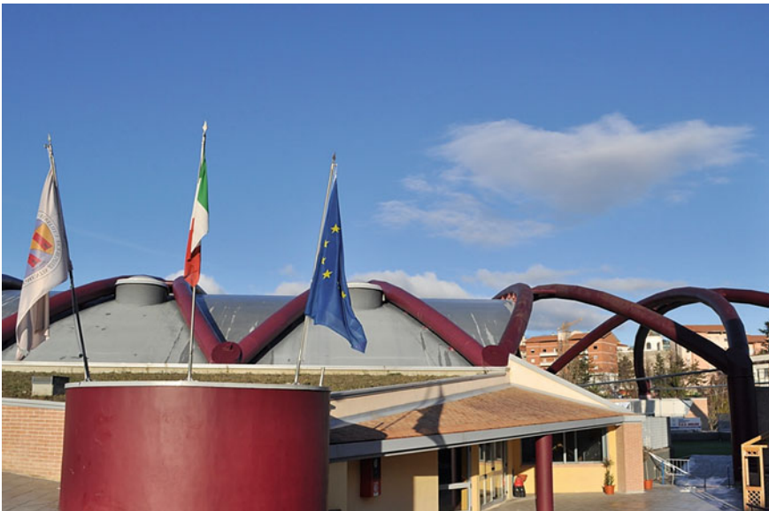
Fig. 1 Outdoor view of the University Sports Hall in Campobasso, Southern Italy, and of the monitored pre-stressed steel cable (on the right in the picture)
