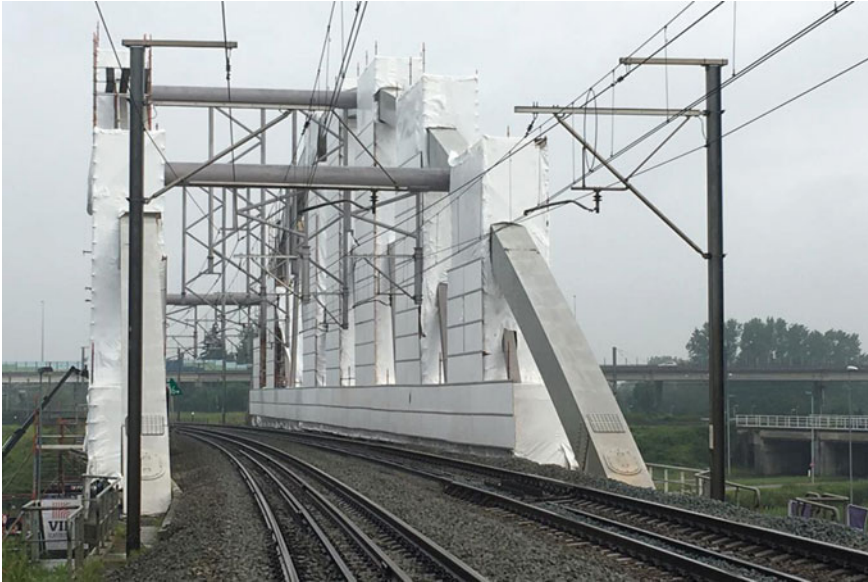
Fig. 11 Bridge with scaffolding during retrofitting
