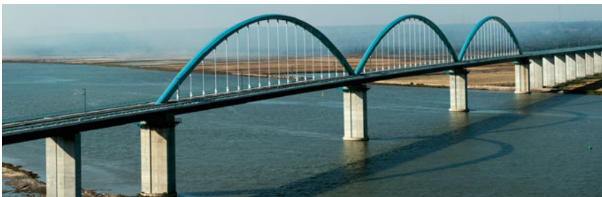
Fig. 3 Overview of the bridge over the Sado River
