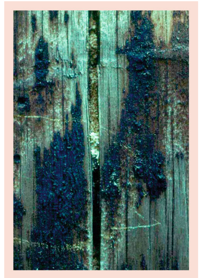
Fig. 4.17 Wood shavings and debris from the interior of a carpenter ant gallery caught in a check at the surface of a preservative treated wood pole. Poles typically are treated with preservatives such that only the outer circumference of the wood (sapwood) is treated. As drying checks develop, carpenter ants will exploit those openings to access the interior untreated wood. The interior wood is then colonized and wood shavings and other debris ejected from the galleries will be found either in piles on the surrounding ground, or more often, caught in cracks and checks such as shown here
