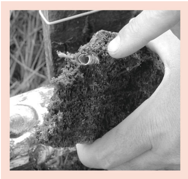
Fig. 4.22 A pine wood plank attacked by both shipworms and gribble. The author's finger (Goodell) points to the calcareous tube extending from the wood, which originally housed the shipworm. This calcareous material lines the entire shipworm gallery inside wood, completely surrounding the animal. The wood surface is fragmented because of the action of gribble
