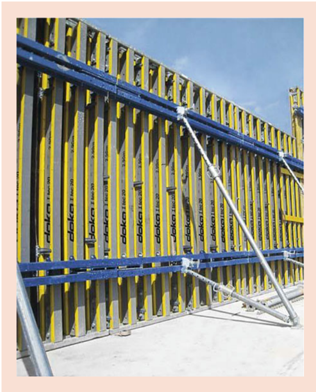
Fig. 35.46 The DOKA formwork system. The vertical standing I-beams (formwork beams) are the main wood-based element in the system
