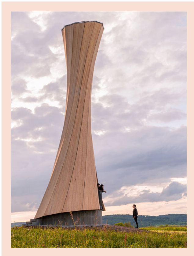
Fig. 35.56 Timber tower made of 14 m-long elements shaped by a self-shaping process to achieve curved timber elements (The Urbach tower in Urbach, Germany). (Photo ICD_ITKE, University of Stuttgart)
