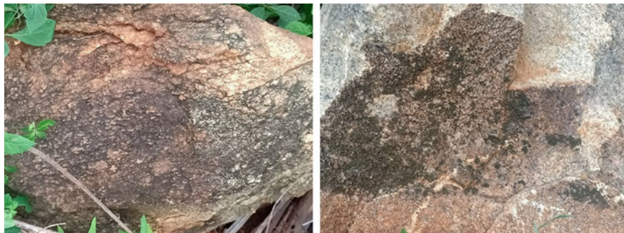
Fig. 3 Disintegration of mineral rock by fungal growth showing cracks
