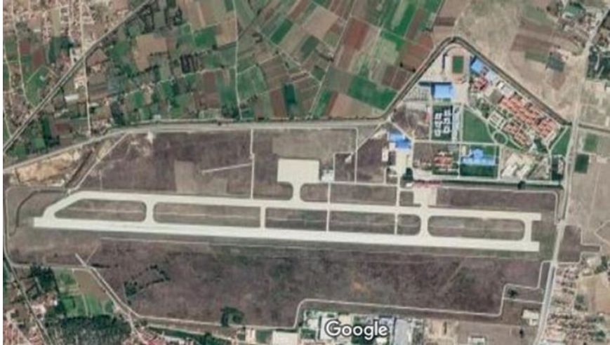
Fig. 3.13 Aerial view of the Eskisehir Hasan Polatkan Airport. (Source: Google)
