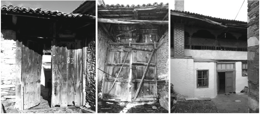
Fig. 2. Entrance gate, from outside and from inside. The materials used are wall made of stone and wood, Photos: Alicja Maciejko, 2020, [3].
