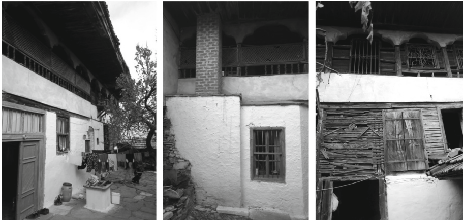
Fig. 3. Construction of walls, view from the courtyard. Photos: Alicja Maciejko, 2020, [3].
