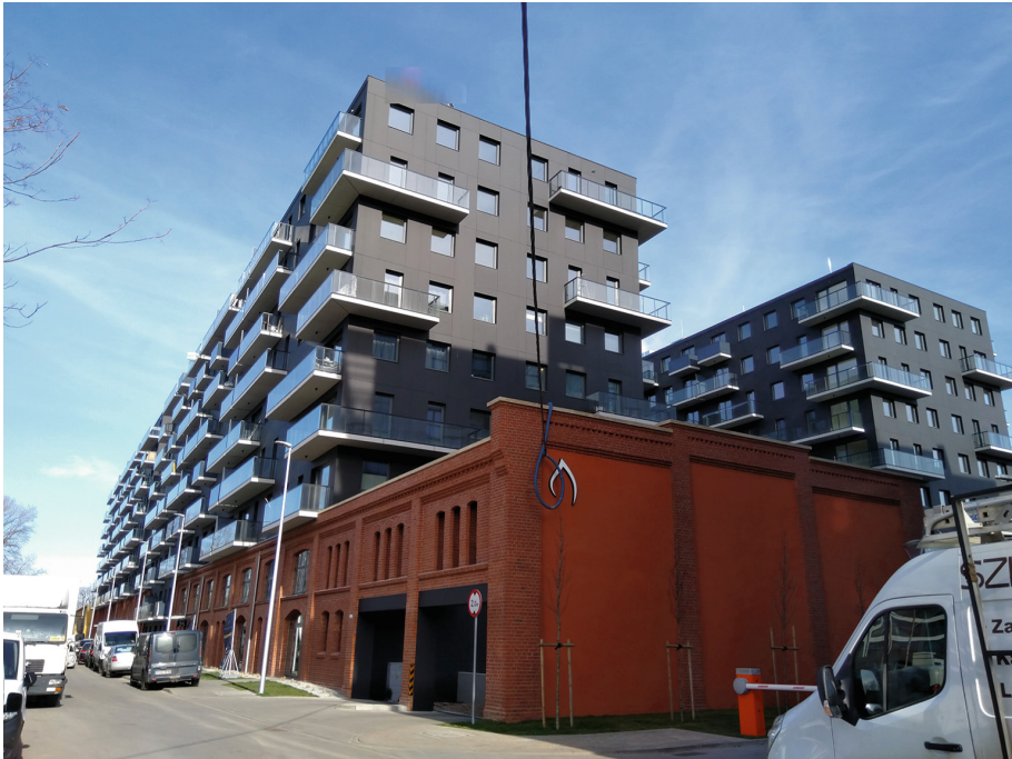
Fig. 2. The expansion of a stable in the artillery barracks in Wrocław (phot. aut.).
