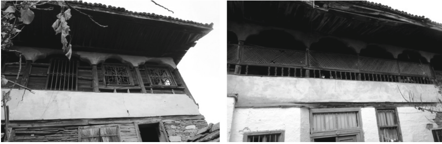
Fig. 4. Entrance wall of the house from the courtyard. Photos: Alicja Maciejko, 2020, [3].
