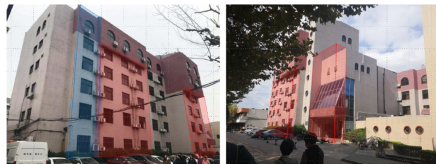
Fig. 2. Status of the south facade
