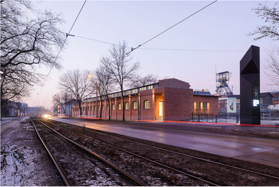
Fig. 1. Coal mine bathhouse Zabrze (Poland). Design: Konior Studio and OVO Grąbczewscy (2014–2015).
