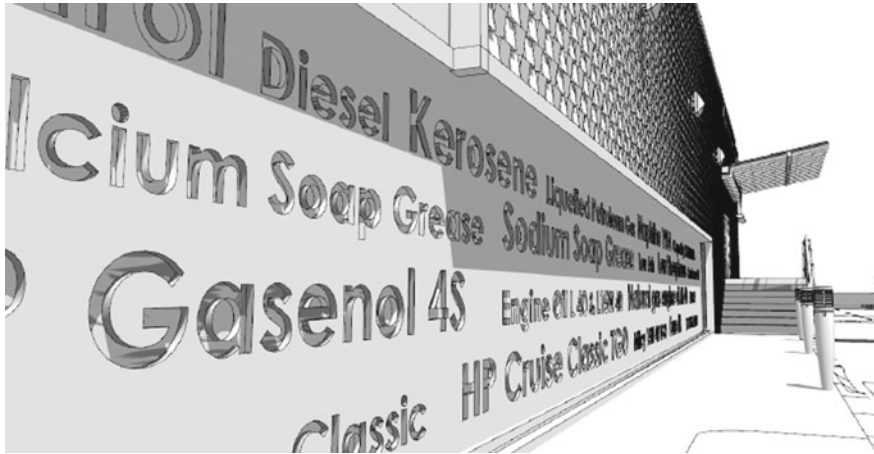
Fig. 7 View of in situ text art in front facade of building
