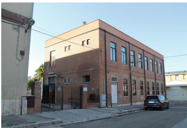
Fig. 14 Street view of the case study school building
