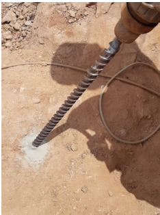
Fig. 2. Drilling the holes
