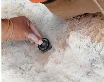
Fig. 6. Placing the plug in the holes
