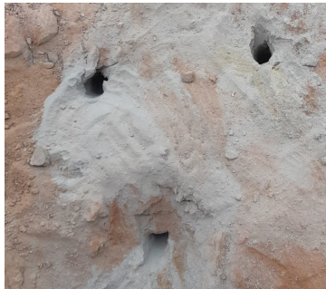
Fig. 3. Drilled holes for test blasting
