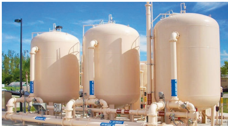
Fig. 8.8 Ion Exchange Filtration setup. (Reprinted with permission of Ion Exchange Filtration, MAA Chem, CC BY 4.0 (Open access), MAA Chem)
