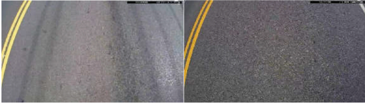
c) Cluster 2 (no apparent cracks)
