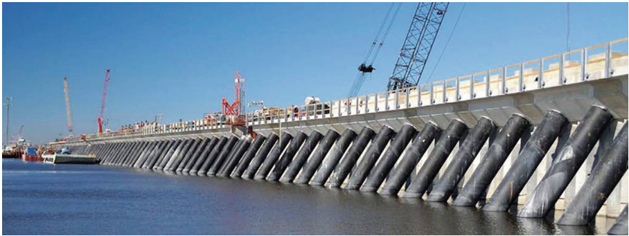
Fig. 1. Floodwall with batter piles during construction
