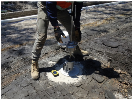
Fig. 6. Light weight deflectometer (LWD) test
