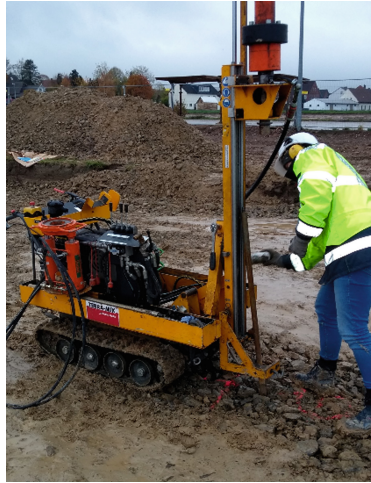
Fig. 12. Performing DPH soundings in the Impulse Compaction field
