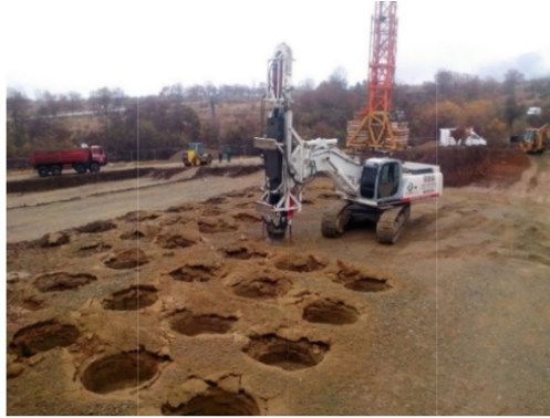
Fig. 5. Resulting craters from the compaction process
