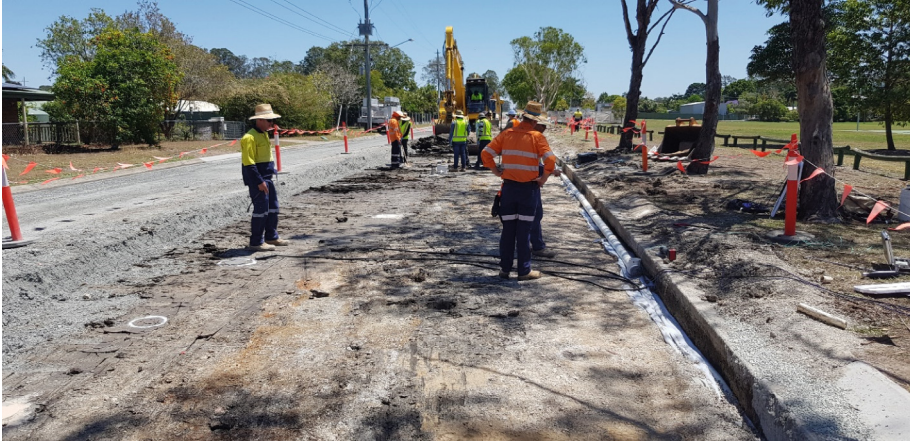
Fig. 3. Excavation of existing pavement in experimental area
