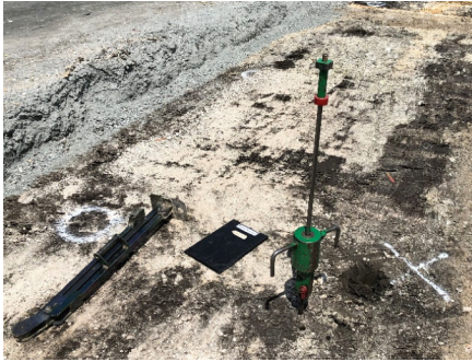
Fig. 4. Dynamic cone penetration (DCP) test
