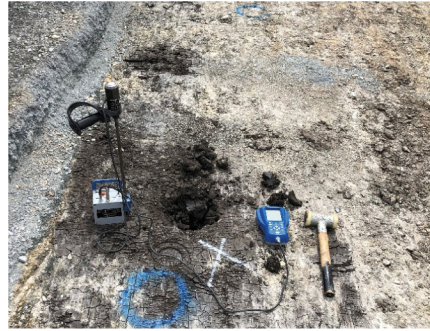
Fig. 5. Variable dynamic cone penetration (PANDA) test
