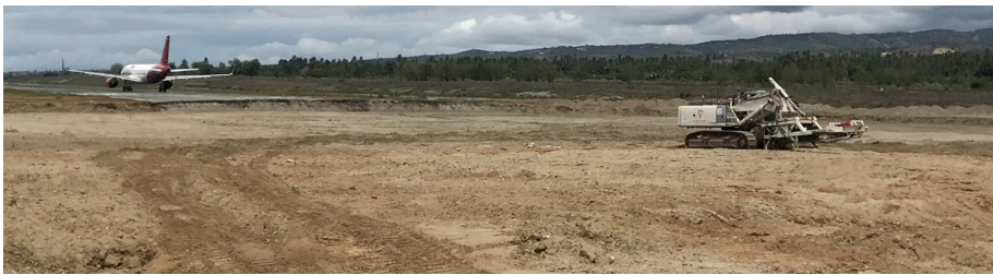
Fig. 21. RIC rig with mast folded down while a plane lands on the Palu airport runway
