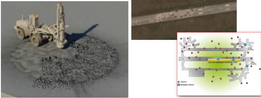
Fig. 4. Port Stanley on Falkland with (repaired) bomb craters (left) and the RRC at work (right) compacting the refilled craters [10].
