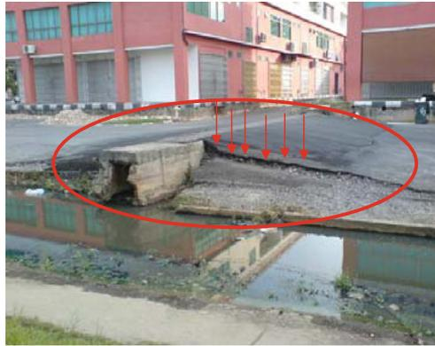
**Fig. 1.** Hazardous settlement of approach road with peat ground subsidence in Sibul, Sarawak, Malaysia (Kolay et al. 2011)
