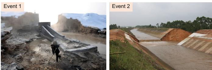
**Fig. 1.** Failures of soil embankments from the field observation (a) Event 1 occurred in Xinjiang, China, February 2013 (Chen 2013) and (b) Event 2 occurred in Guangdong, China, May 2014 (Yu 2014).
